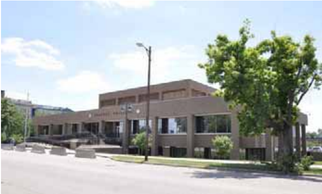
U.S. General Services Administration Federal Office Building
